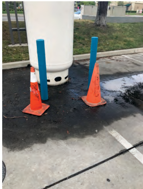
PAINT BUMPER POLES NEAR TANK SAFETY YELLOW. NO TOUCH TANK.
