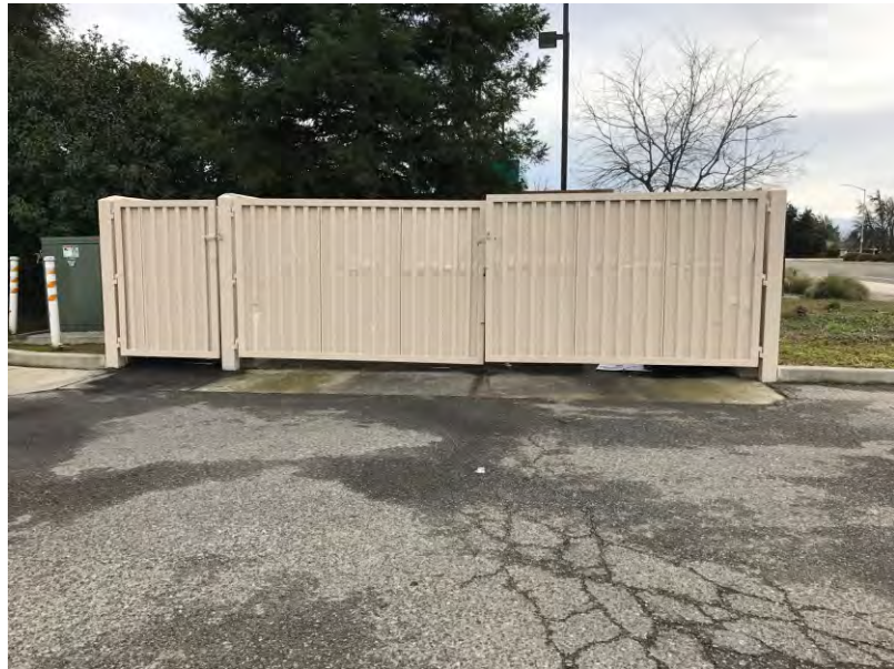
PAINT TRASH ENCLOSURE VALERO SAND. PAINT TRASH ENCLOSURE DOORS VALERO LIGHT GRAY. NO TOUCH BUMPER POLES NEAR ELECTRICAL BOX WITH REFLECTIVE STRIPES.
